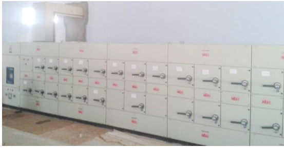
Fig.5. New MV Panel
