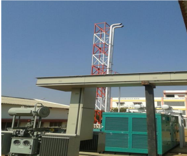
Fig. 1. Flue Gas Emission Outlet (Control Pollution Control Board Norms)
